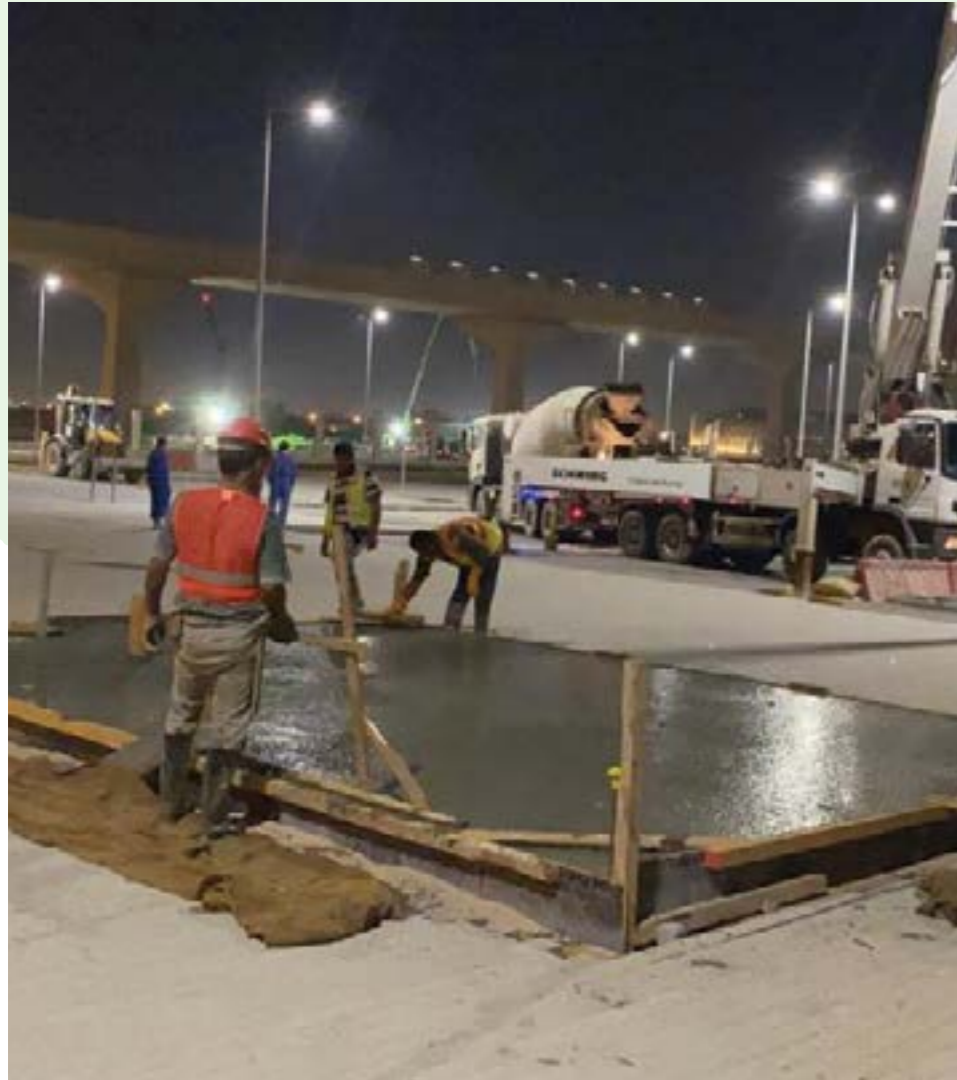
First step we design and calculate strong base foundation to accommodate desired design and final product we execute with high level of standards.
